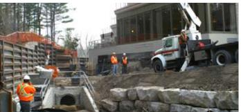
To achieve this goal, the first step was finding a way to stabilize the bank in an aesthetic way. To provide enough space for the yard, a wall needed to be built directly on the property line. However, a conservation area was adjacent to the property, making a geogrid-reinforced or tiered wall impossible.
